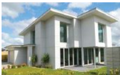
The Chinese government has developed energy codes for buildings to reduce pollution
