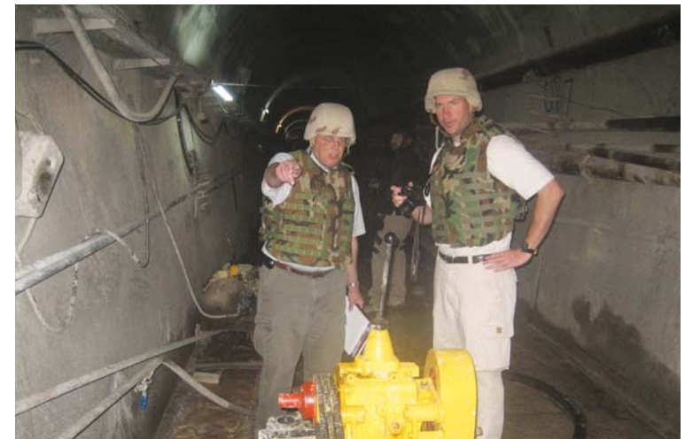
Members of SIGIR team inspect work at Mosul Dam.
