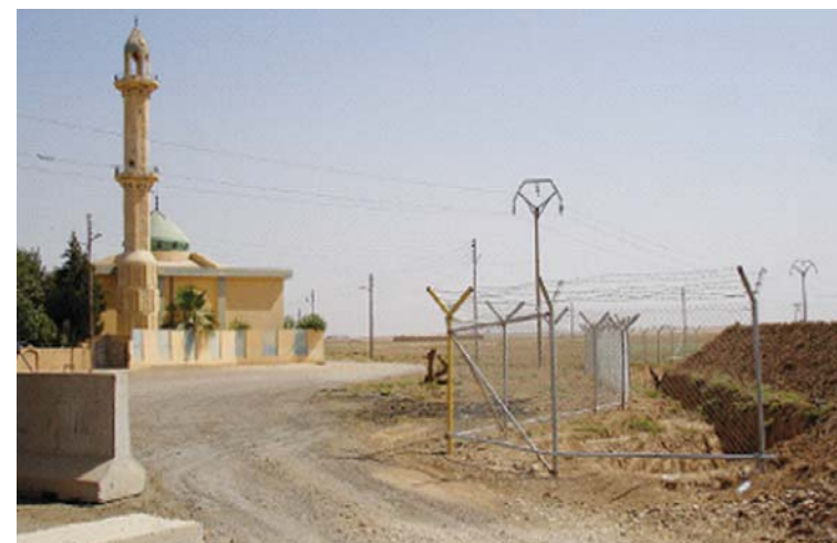
Under the ESF-funded Infrastructure Security Program, the United States supported construction of secured corridors to protect oil pipelines from insurgent attacks. The program contributed to an almost 12-fold increase in northern exports from 2006 to 2008.
