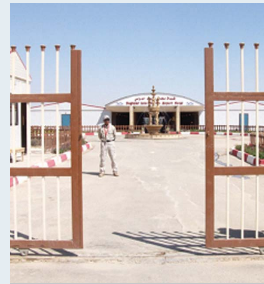
The United States spent $4.2 million in CERP funds to build the Caravan Hotel at Baghdad International Airport.
