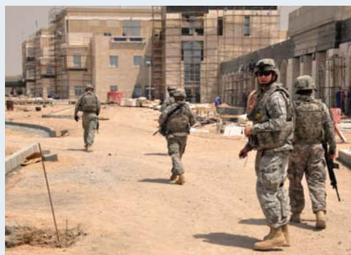
U.S. soldiers look over the grounds of the Basrah Children's Hospital under construction in May 2009. (U.S. Army photo)
