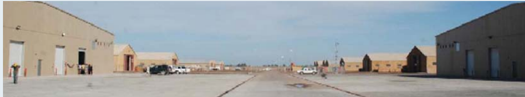
The Depot Distribution Central Operation storage facilities at Camp Taji was completed in November 2010. (USACE photo)
